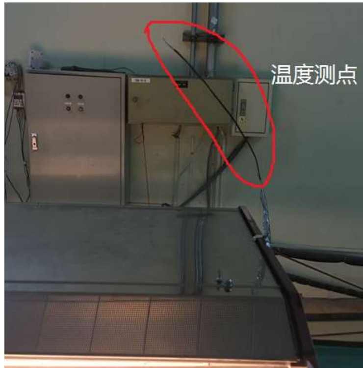
Figure 1-3 Layout of ambient temperature measurement points
