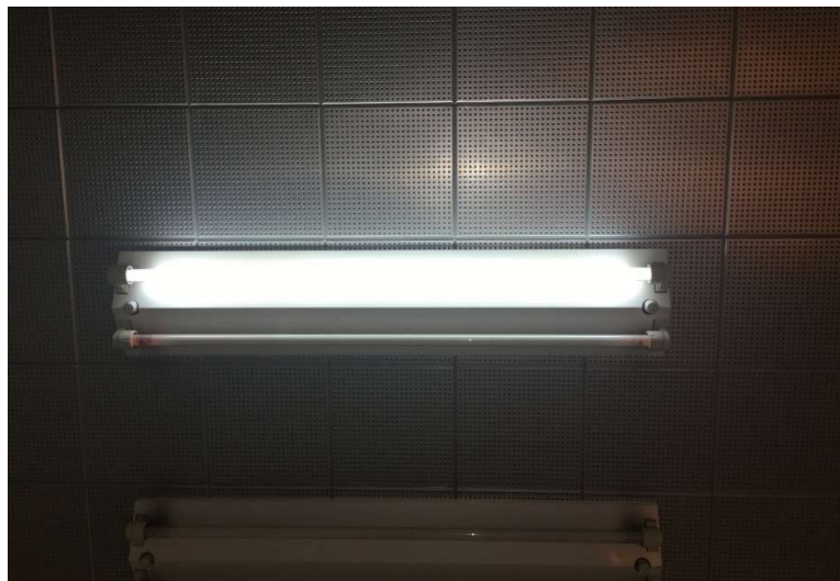
Fig. 1-1 Laboratory air supply wall
